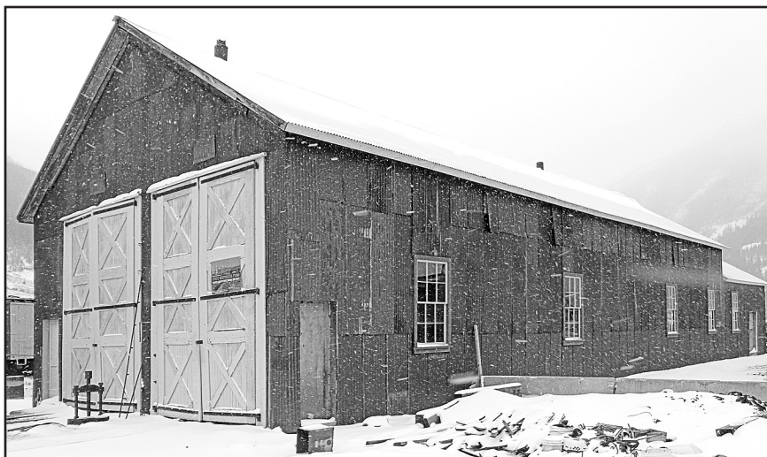
Restoration of the engine house with salvaged corrugated metal sheathing on the walls and new window sashes. – Photo © 2019 Jerry Hoffer.
